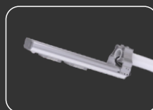
Arm lamp installation
